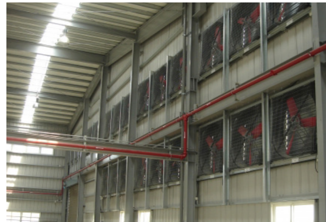
Ventilation in factories in Asia
