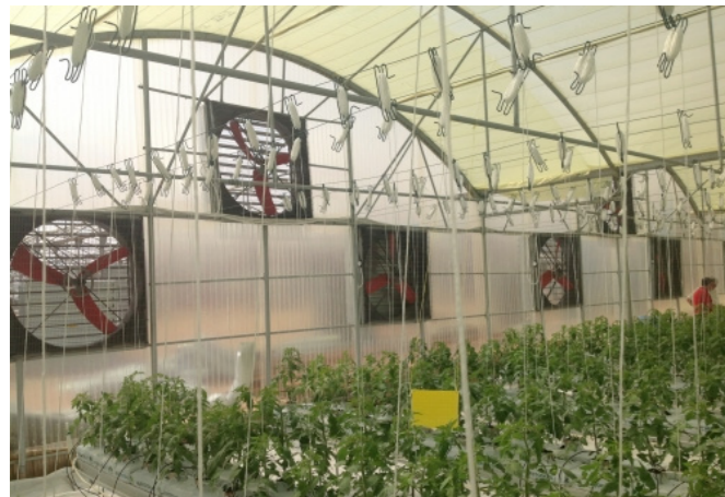
Fans applied in a tomato greenhouse in the Middle East
